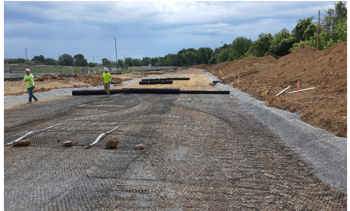
Geogrids enhance soil separation and stabilization qualities.
